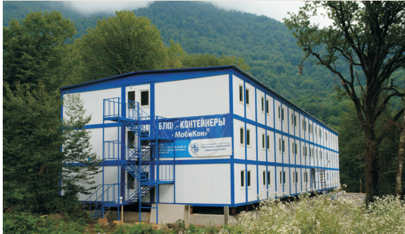
Figure 3. The prefabricated demountable three-storey building structure composed of block-containers (the city of Sochi)
