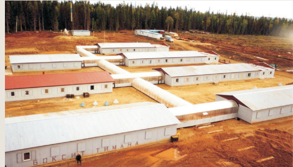
Figure 4. Camp for shift work with pedestrian tunnels (square is 1880 sq m) in the Komi Republic, Sredne-Timanski mine
